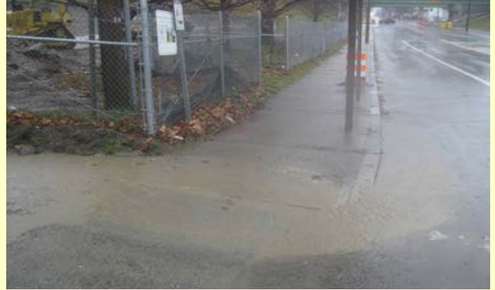
Polluted stormwater runoff due to lack of adequate Control Measures.
