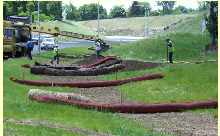
Compost filter sock used for velocity dissipation and sediment control.
