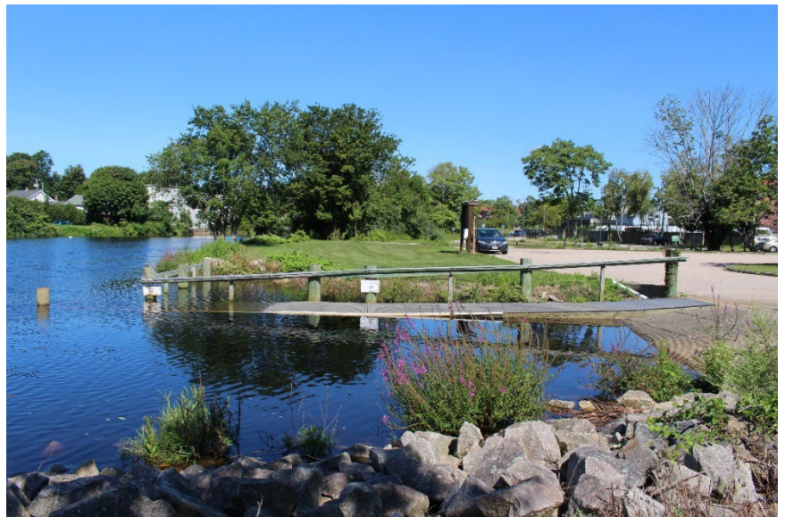
The new Main Street boat ramp will have the same footprint as the existing ramp and feature new adjacent floating docks to replace the deteriorating fixed-dock system.
