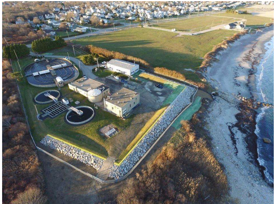
The Town of Narragansett obtained a matching, $650,000 resilience grant in 2020 to fortify the Scarborough wastewater treatment plant against more intense coastal storms.
