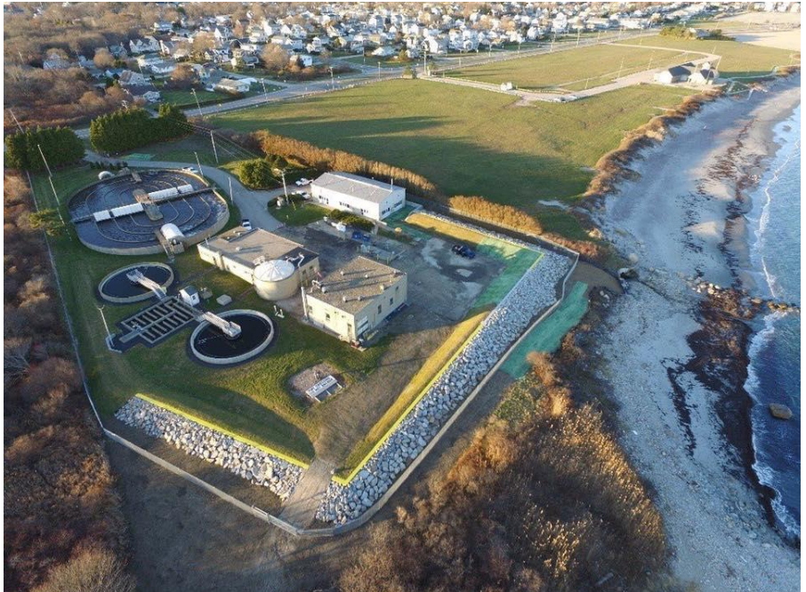
The Town of Narragansett obtained a matching, $650,000 resilience grant in 2020 to fortify the Scarborough wastewater treatment plant against more intense coastal storms.
